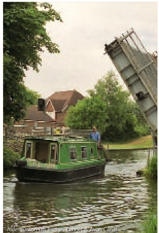
Aldermaston Lift Bridge, Kennet & Avon Canal
